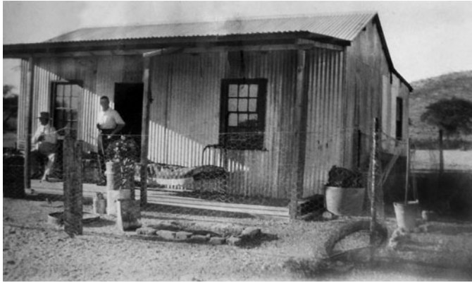
Figure 1. The home of J.J. Davis, railway worker, on the outskirts of Usakos, 1932. A simple wood construction with nailed walls of corrugated iron and no sanitary installations (except a makeshift outdoor bucket latrine), the house was threatened with removal because of its quality and proximity to the African location. (NAN: SWAA-1831-A382/14)
