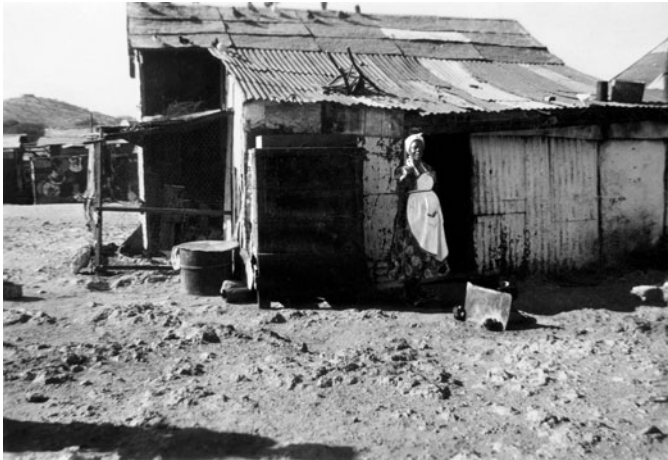
Figure 3. Cecilie Geises in front of her mother's house (wooden construction with corrugated iron walls and roof), Usakos old location, 1950s. (Private collection, Cecilie Geises)
