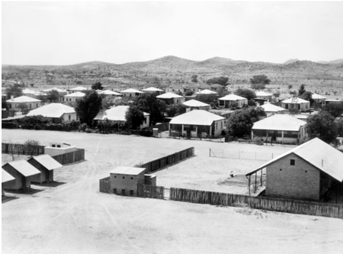
Figure 2. View of an early South African Railways housing scheme in Usakos, built in the 1930s. Similar schemes of plastered brick buildings were realised, especially after the Second World War. (Transnamib Railway Museum, Antonie Swanepool Collection)
