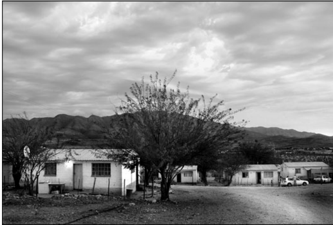
Figure 5. Some of the NE 51/6 houses built in the early 1960s in the Hakhaseb township of Usakos; in the background on the right, the town centre of Usakos, with the area of the old location in between. (Photograph: Paul Grendon, 2013)
